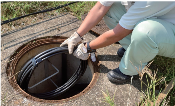
Fig. 9. View of installation in a handhole.
