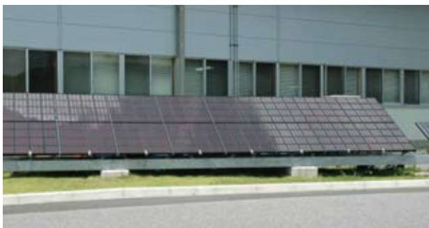
Fig. 4. Outdoor operation test of DSC module panels.
