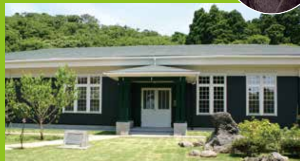
Main Building of Oshima Fujikura Gakuen
