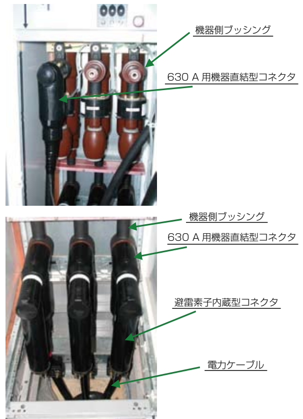
図7 630 A 用機器直結型コネクタの接続状況(例) Fig. 7. Connection status of the separable connectors for 630 A (cases).
