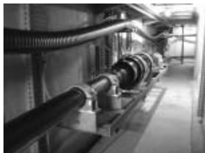
図9 PQ長期試験状況 (PJ) Photograph of PQ long-term test line
