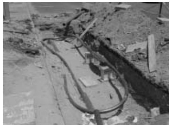
図12 通信ケーブル接続状況 Straight through joint for pilot cable
