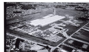
Suzuka Plant upon completion
