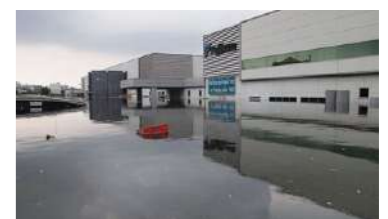
Flooded plant in Thailand
