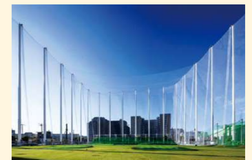
New safety net poles updated to prevent wind damage
