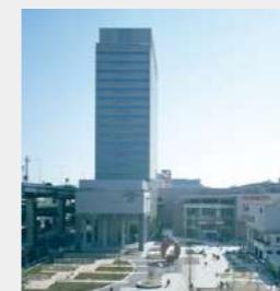
Fukagawa Gatharia redevelopment project
