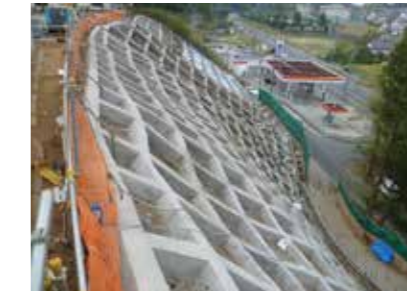
Slope face construction at Sakura Works
