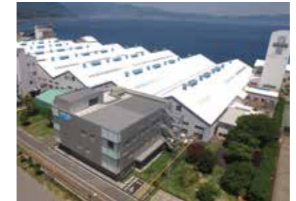
Tsunami evacuation tower at Nishi Nippon Electric Wire & Cable
