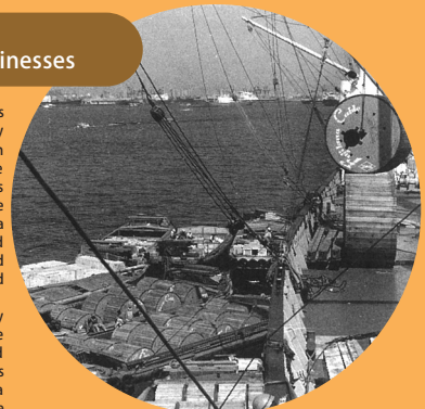
Loading of export OF cables into ship
