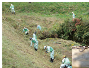
Cutting grass on slope
