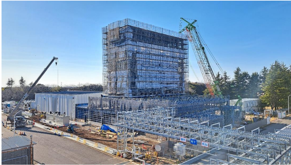
▼ New factory under construction
